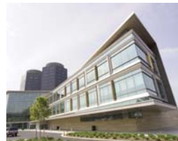
Phase I of Stony Brook University Medical Center's Major Modernization project was recently completed.
