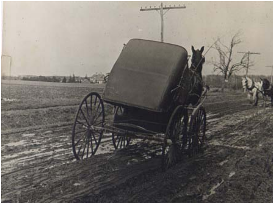
Figure 1: Melville Road, then called Farmingdale Road, reflects the rural nature of undeveloped Long Island in this pre-1912 image. The horse and carriage are having difficulty traversing the muddy road. The agricultural school would be built on land to the north. — All images in this article are courtesy of the SUNY Farmingdale College Archives.
