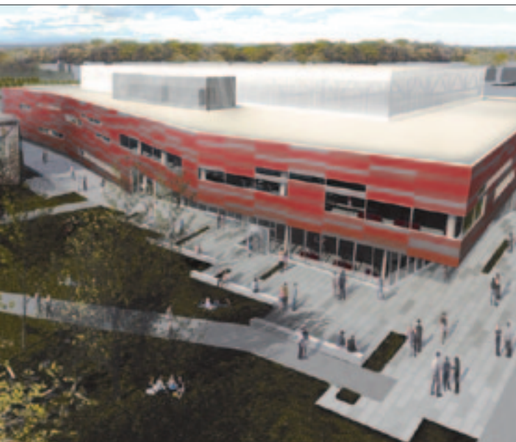
The New Student Recreation Center.
